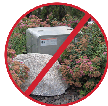
BAD EXAMPLE: Not accessible to utility workers
