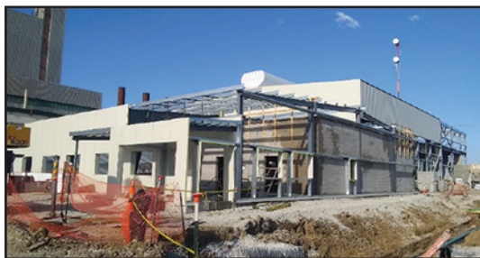
Work at Summit Lake Generating Station in Creston moves forward.
