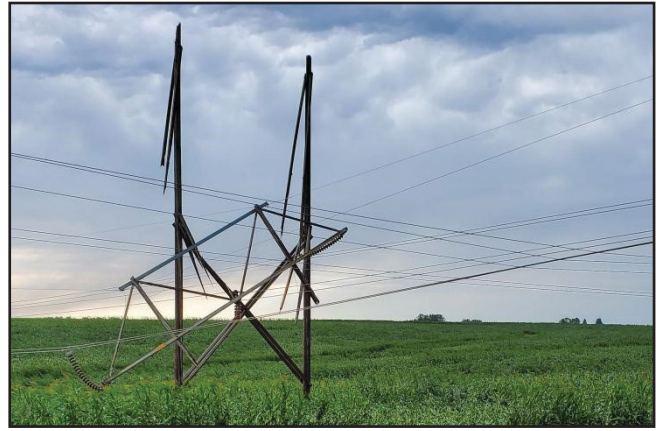
Above: Strong winds took down part of a transmission line owned by MidAmerican Energy. Photo by PCEA Journeyman Lineman Matt Ainsworth.
